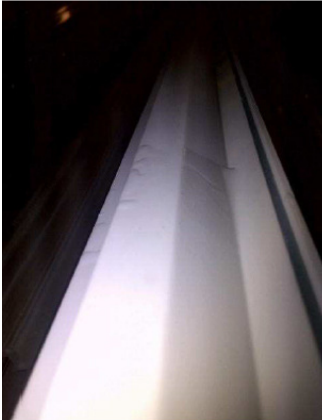
Water Test Photo #1 – Prep Pass
